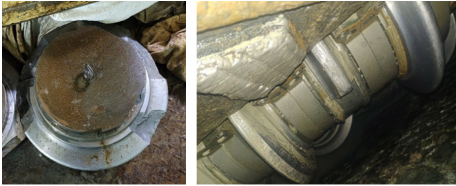
Fig. 3. Fracture cases of disc cutters at utility cable tunnel C
